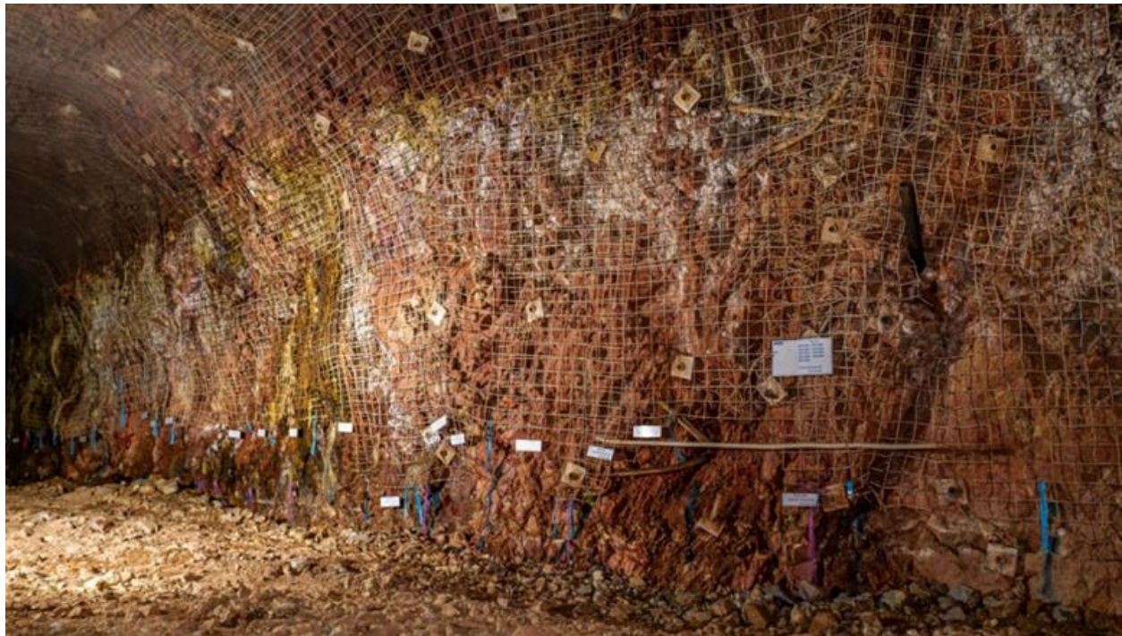
Figure 7-18: View of Veins VN-05, 06, 07 in the North Ramp Underground Workings
